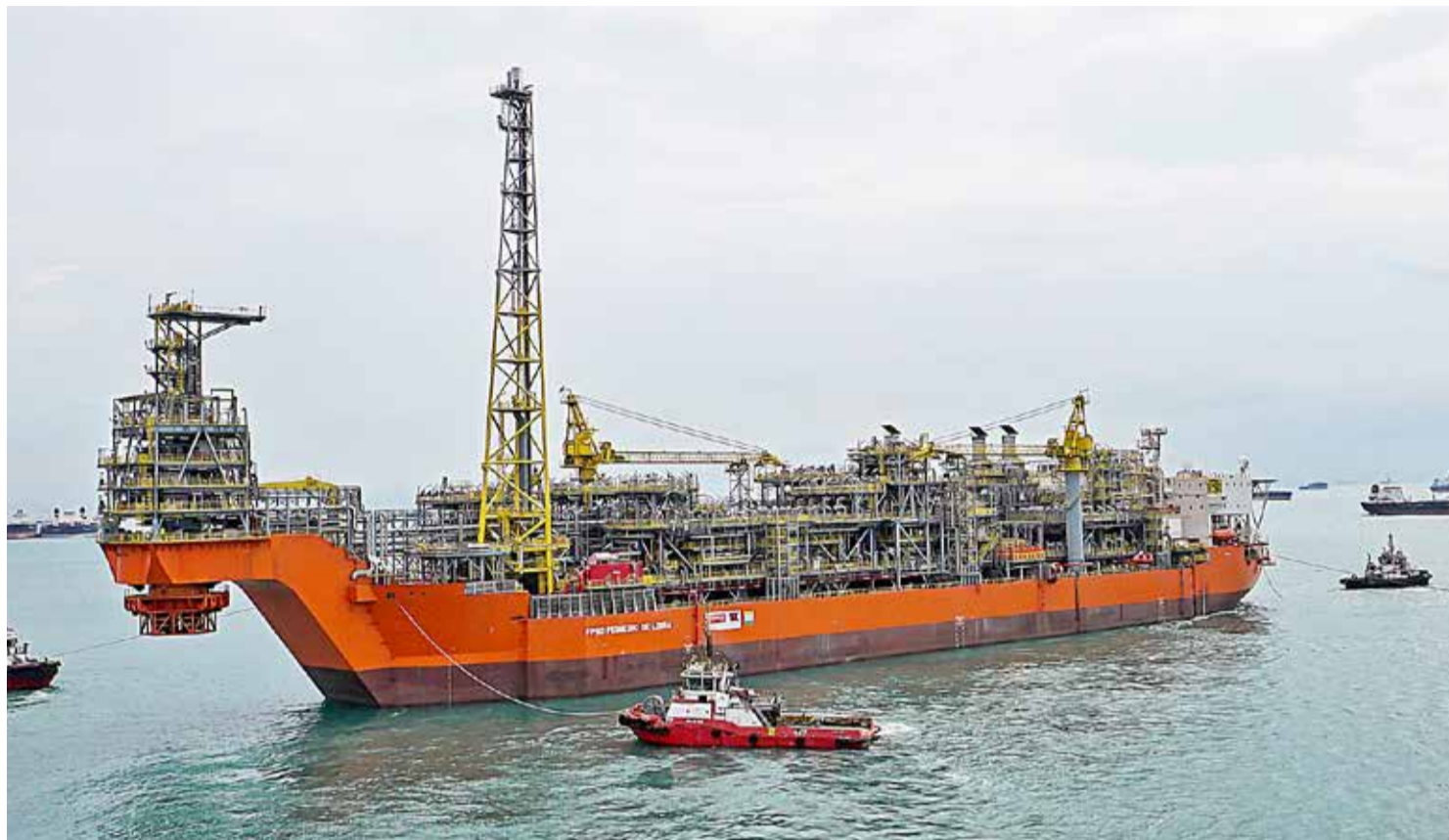
Testing ground: Petrobras is using eight-inch diameter lines to produce from the Mero extended well test with the Pioneiro de Libra FPSO
